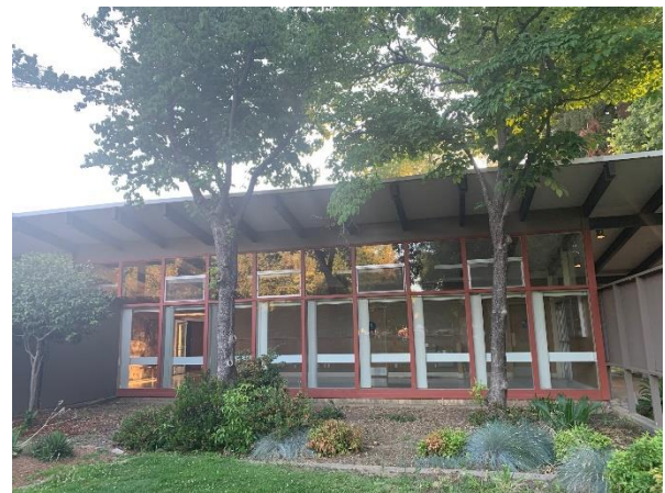
Above: Bed outside entrance hall.
